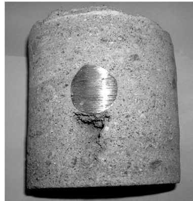
Dry-mix shotcrete, #8 bar, one important void directly behind rebar, smaller than 1/4 dept and 3/4 in long.
