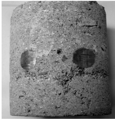
Dry-mix shotcrete, #4 bar, sand lenses.
